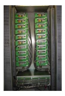
The split core CT is a single channel current input, where the CT secondary cable goes through the center of the split core and the output will be wired directly to TESLA's analog input. The benefit of using the split core CT is that it does not require a power outage or disconnection of the CT during the installation. The picture below shows a typical split core CT installation. A separate split core CT mounting bracket is also available to have the CTs DIN rail mounted.
