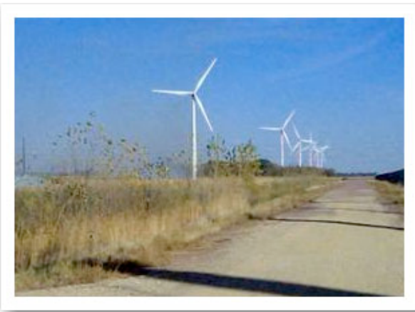
Wind farm located in Midwest USA is site of first S-PRO installation.
