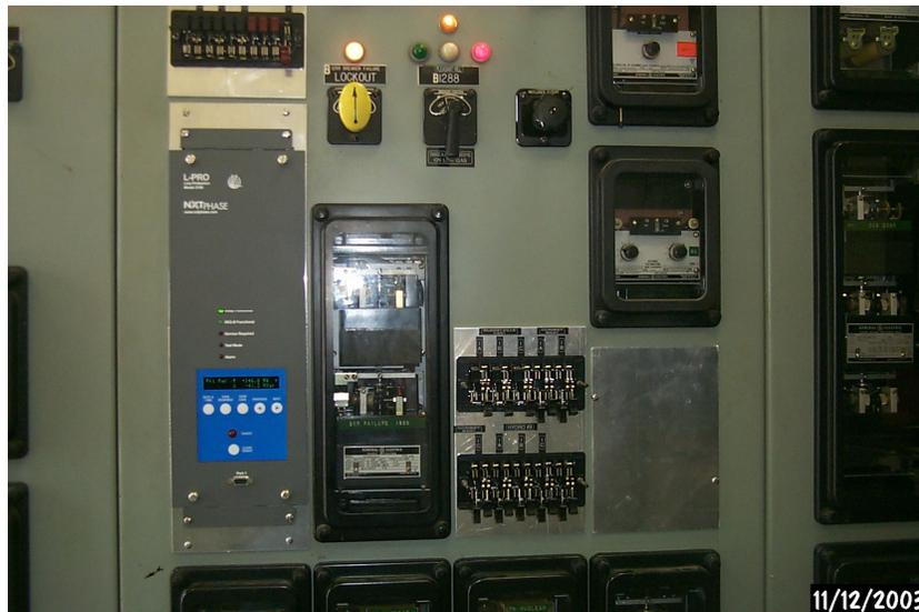
Figure 7: Relay installed in protection panel
